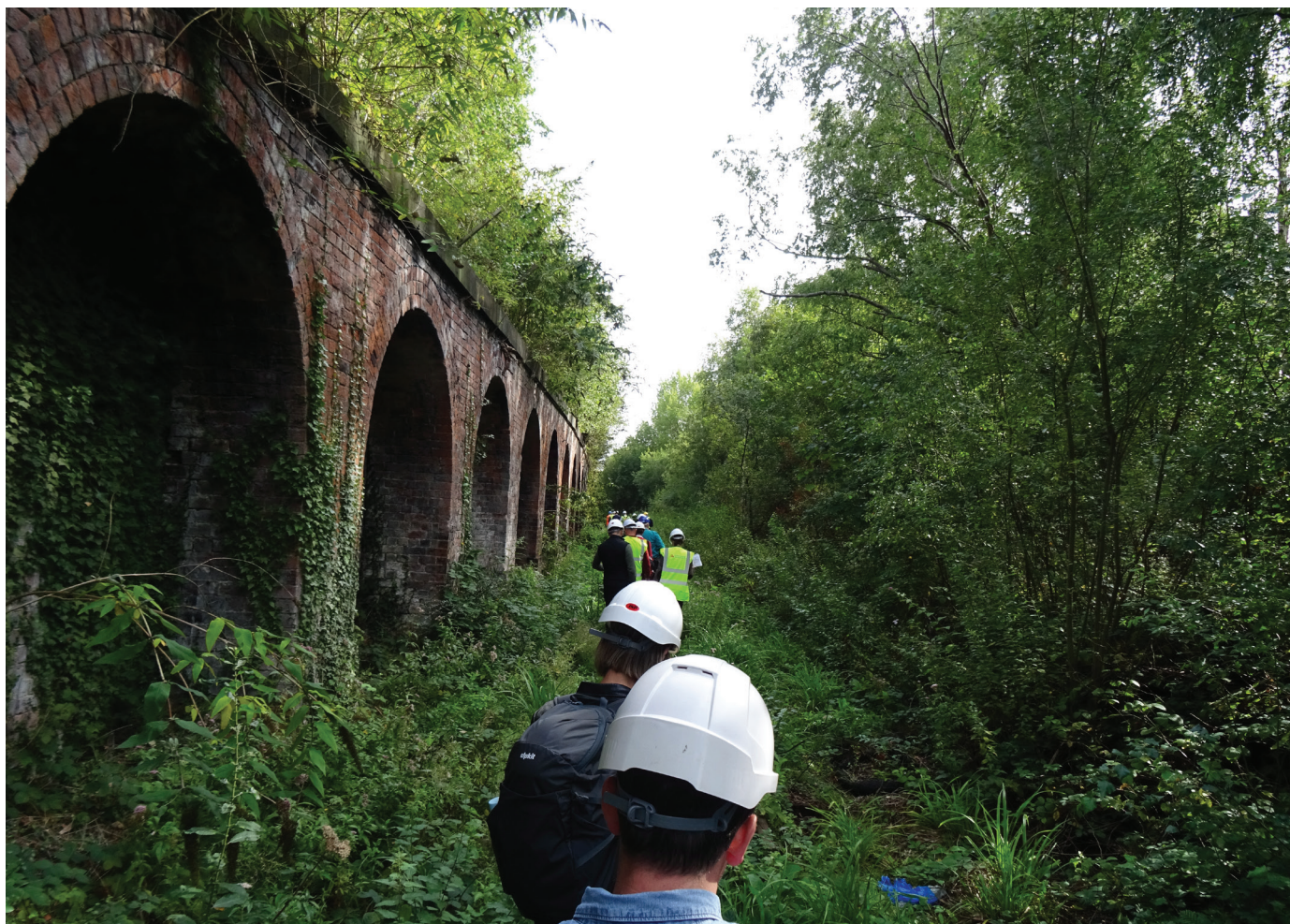
Dock Branch cutting
